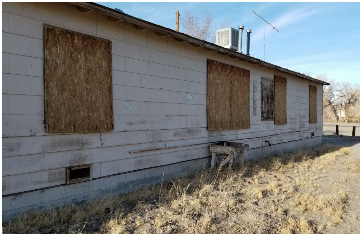
Figure 6. Far east side of the old school showing boarded windows and deteriorated paint.
